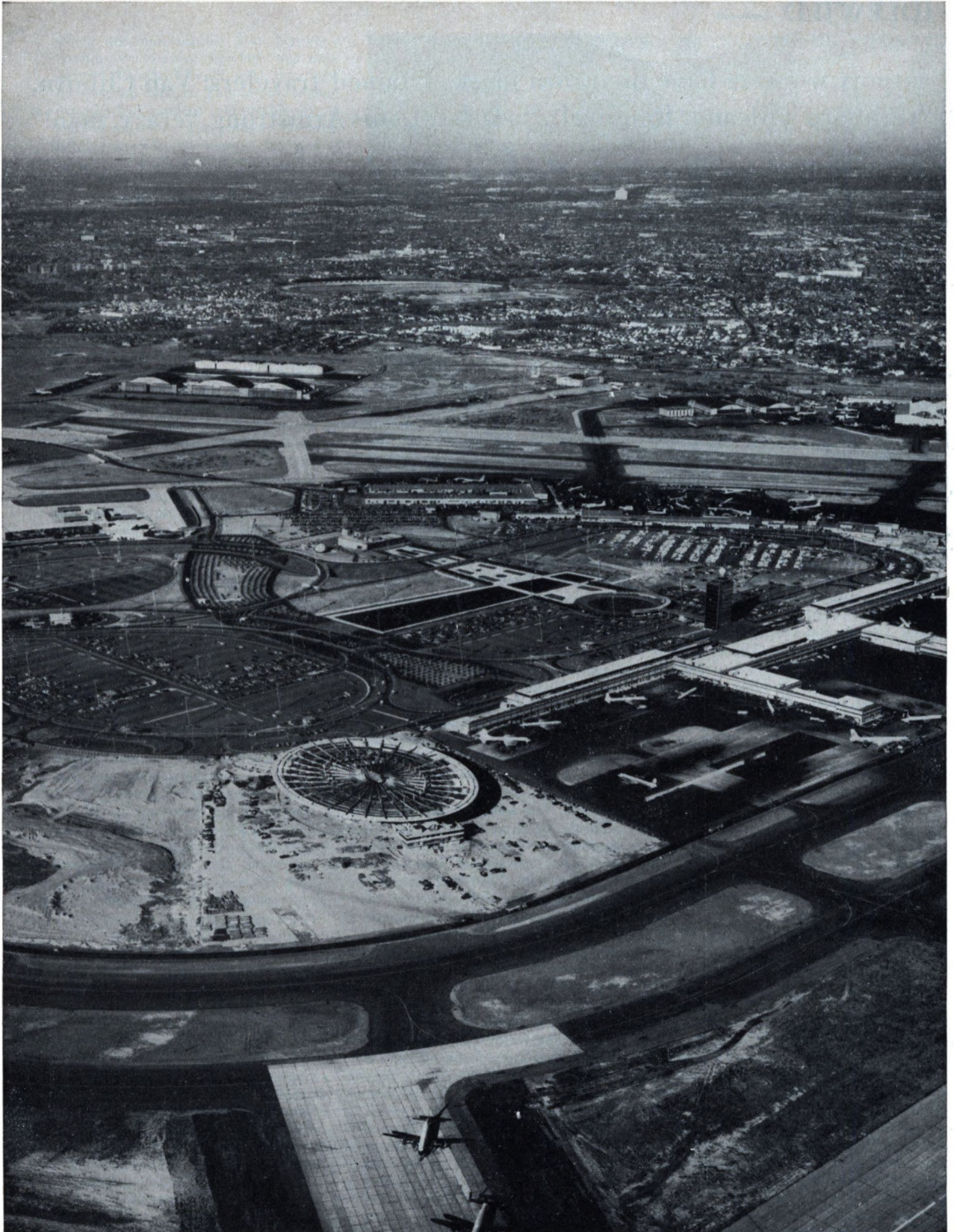
JETS-EYE VIEW of world's busiest air terminal shows cluster of new buildings, mammoth runways where seven
